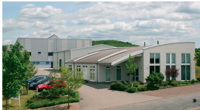
The Miehlen/D facility.
